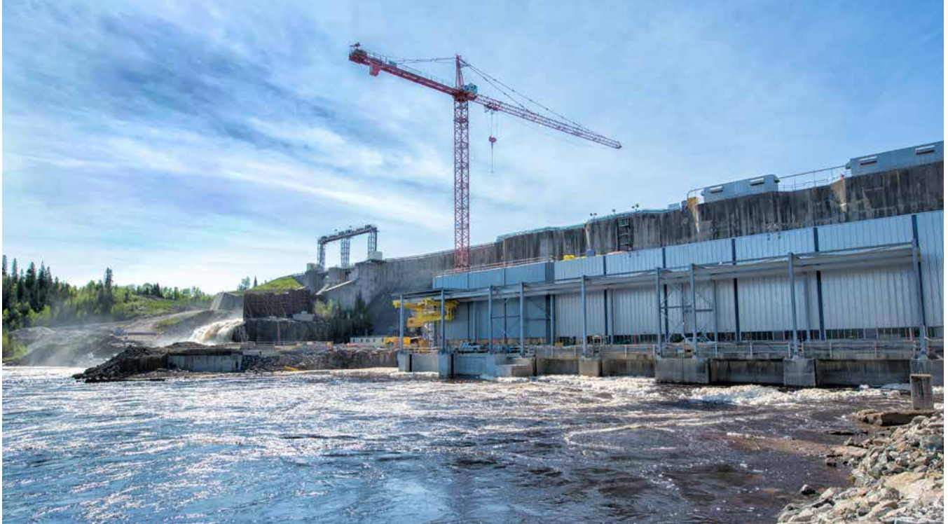
Lower Mattagami, Kipling GS construction
